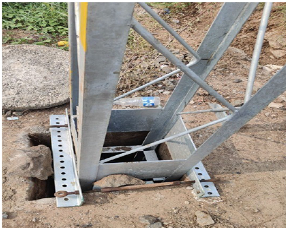
Arrangement for securing ungrouted Mast/Portal upright
