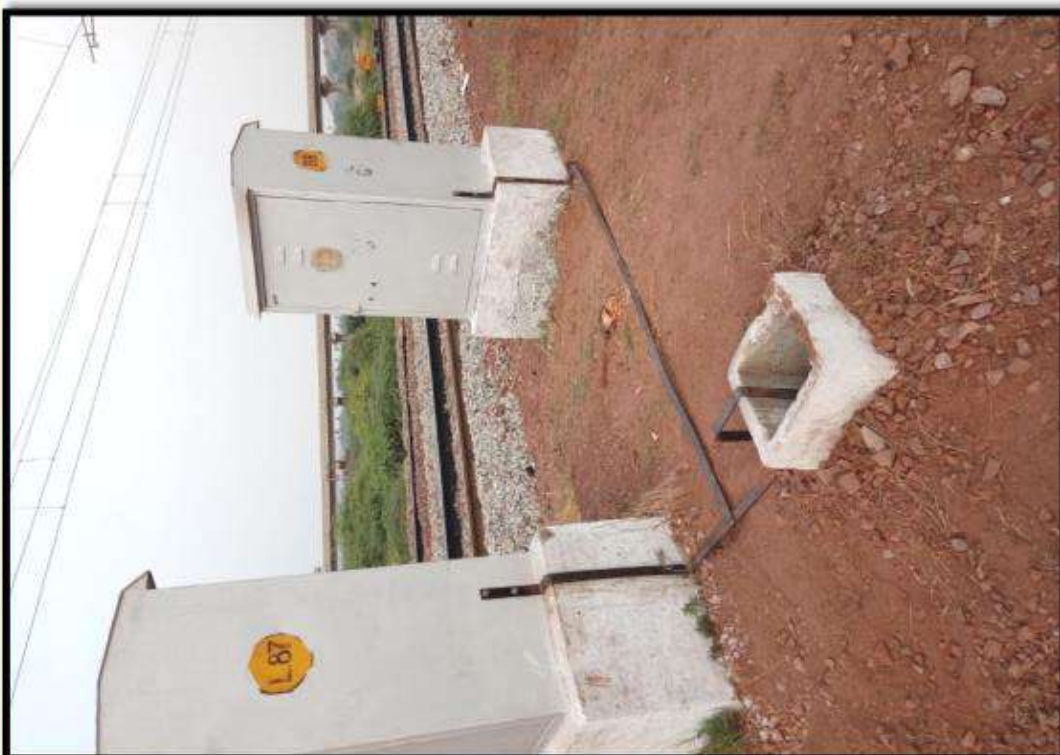
MS FLAT EARTHING AT LOCATION BOXES
