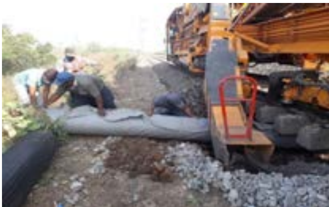
Fig-10.3(a): Insertion of Material under BCM
