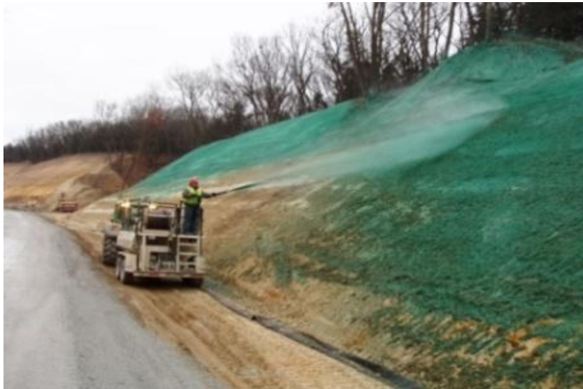
Fig-8.5 Figure showing Hydro-seeding/hydro-mulching on slope
