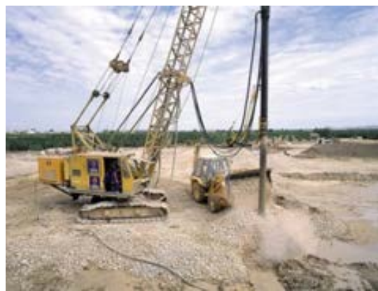
Fig- 2.4: Ground improvement using stone column
