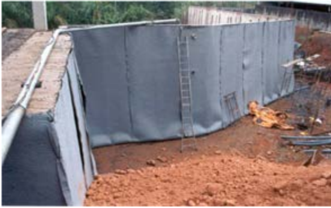
Fig 4.19: Installation of Geocomposite Drain
