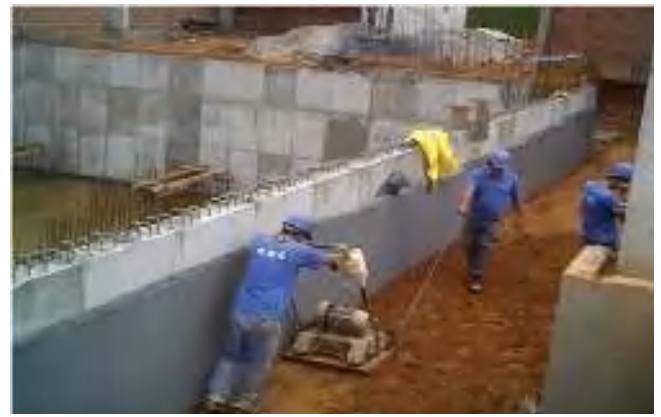
Fig 4.19: Installation of Geocomposite Drain
