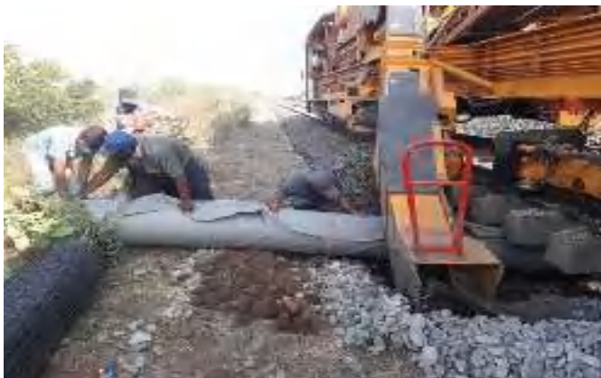
Fig-10.3(a): Insertion of Material under BCM
