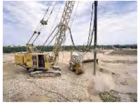
Fig- 2.4: Ground improvement using stone column
