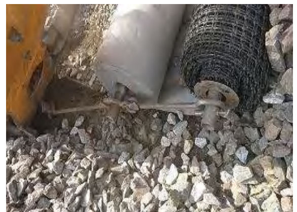
Fig-10.3(b): Linking of Rolls to BCM
