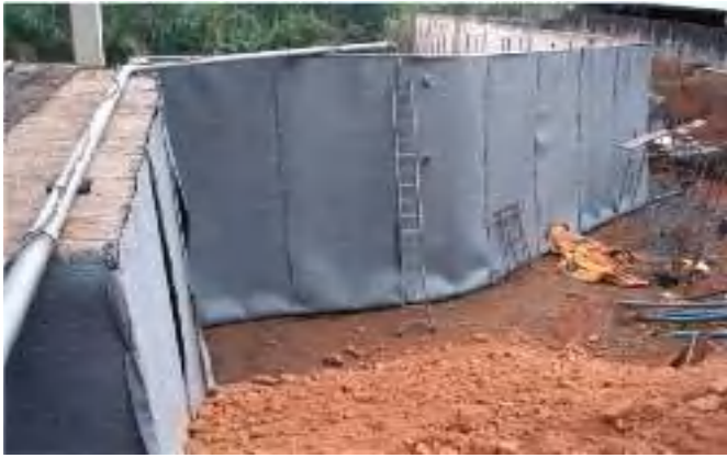
Fig 4.19: Installation of Geocomposite Drain
