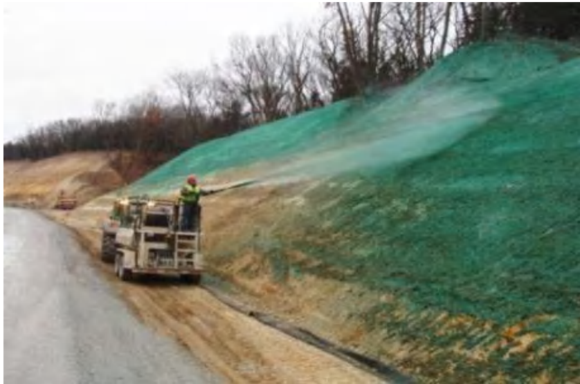
Fig-8.5 Figure showing Hydro-seeding/hydro-mulching on slope
