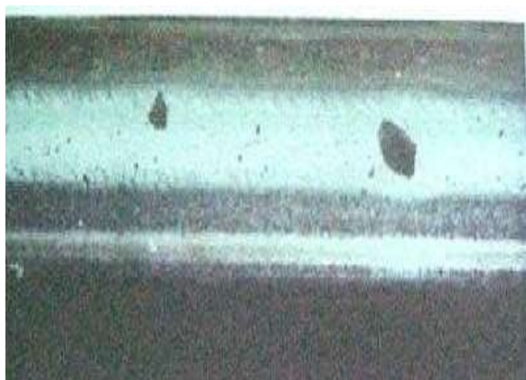
FIG. 48 : 301 - DAMAGE TO RAIL BY BRUSHING OR ARCING
