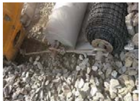
Fig-10.3(b): Linking of Rolls to BCM
