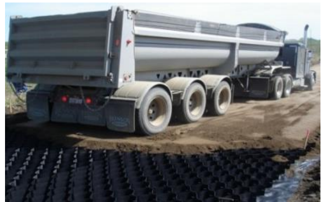
Fig-2.6(b): Geocell and it's applications
