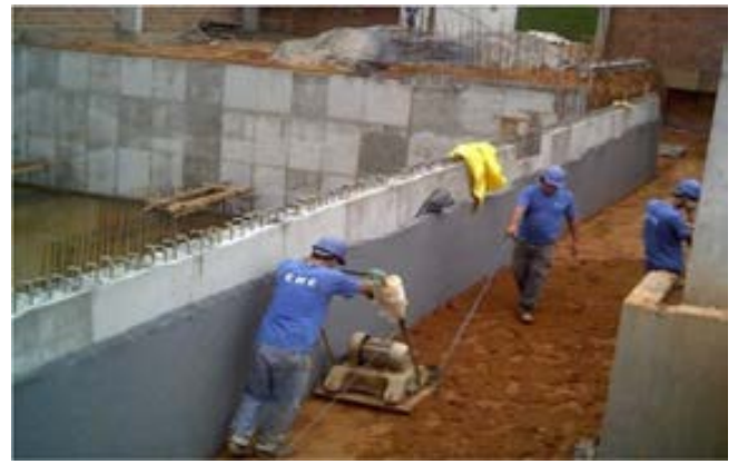
Fig 4.19: Installation of Geocomposite Drain
