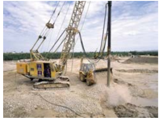
Fig- 2.4: Ground improvement using stone column
