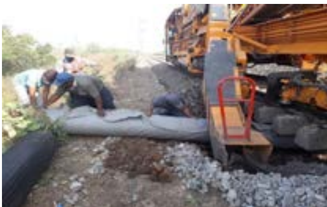
Fig-10.3(a): Insertion of Material under BCM
