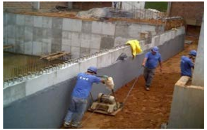
Fig 4.19: Installation of Geocomposite Drain
