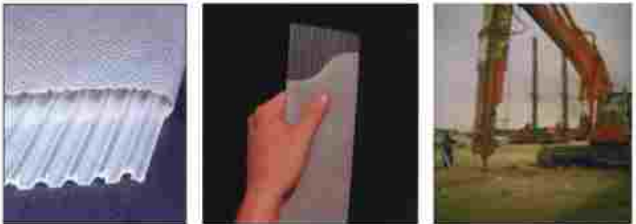
Fig-2.7: PVDs and their Installation
