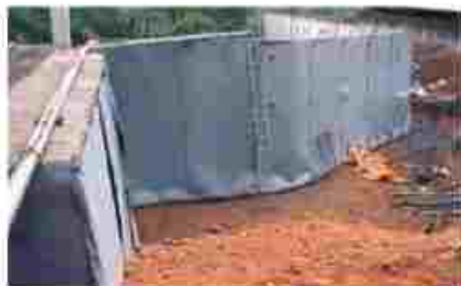
Fig 4.19: Installation of Geocomposite Drain
