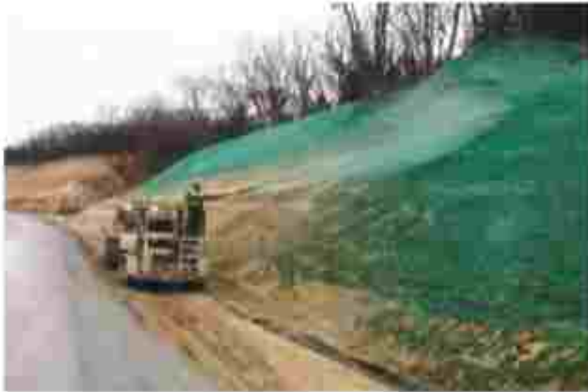
Fig-8.5 Figure showing Hydro-seeding/hydro-mulching on slope
