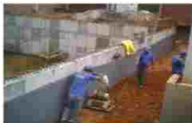
Fig 4.19: Installation of Geocomposite Drain
