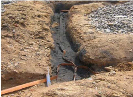
Figure 4 : Interlinking of earth pits using copper tape
