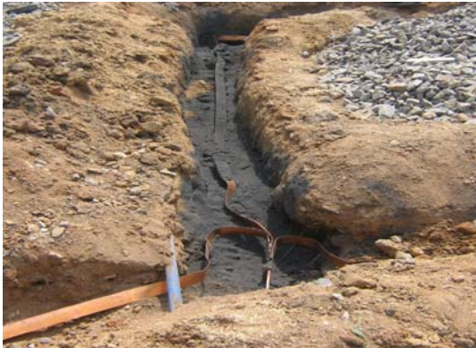
Figure 4 : Interlinking of earth pits using copper tape
