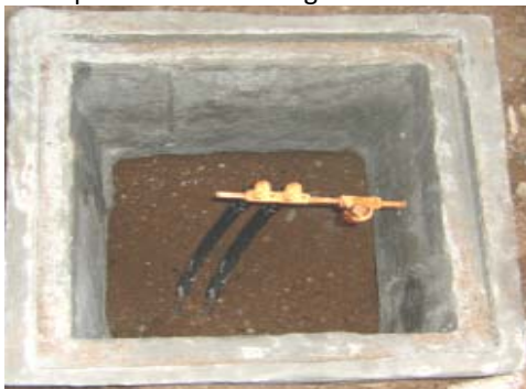
Figure 5: Inspection chamber
