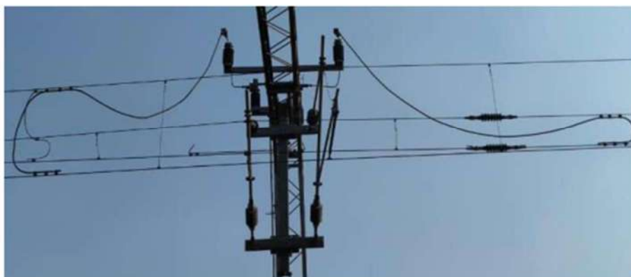
ISOLATOR JUMPER CONNECTION WITH 3PG
