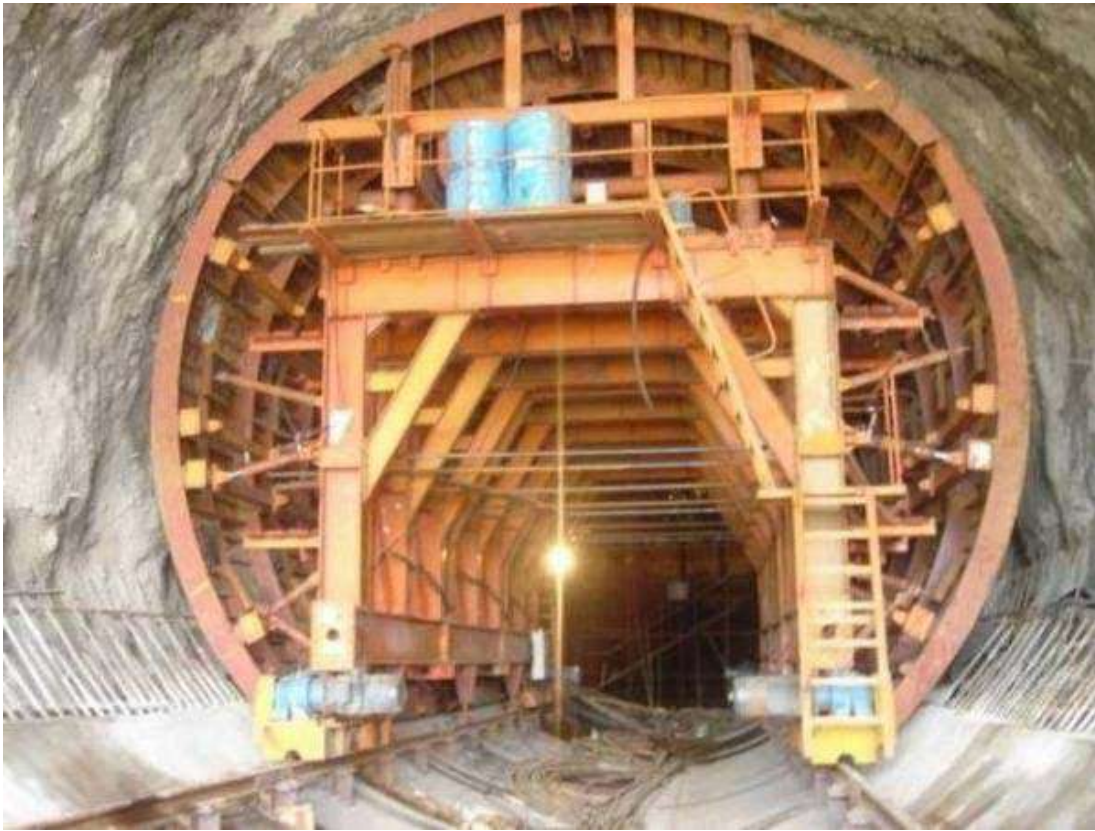
Figure 17: Concrete lining using Gantry shutter
