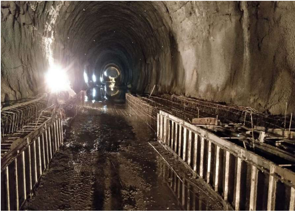
Figure 16: R/F and Shuttering for Kerb concrete
