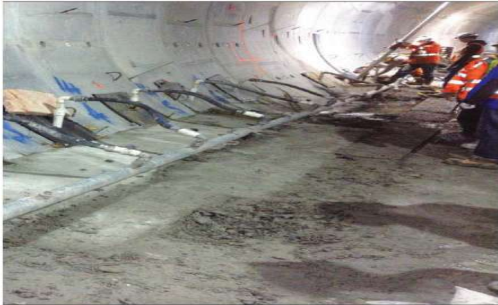
Figure 20: Dewatering process during construction
