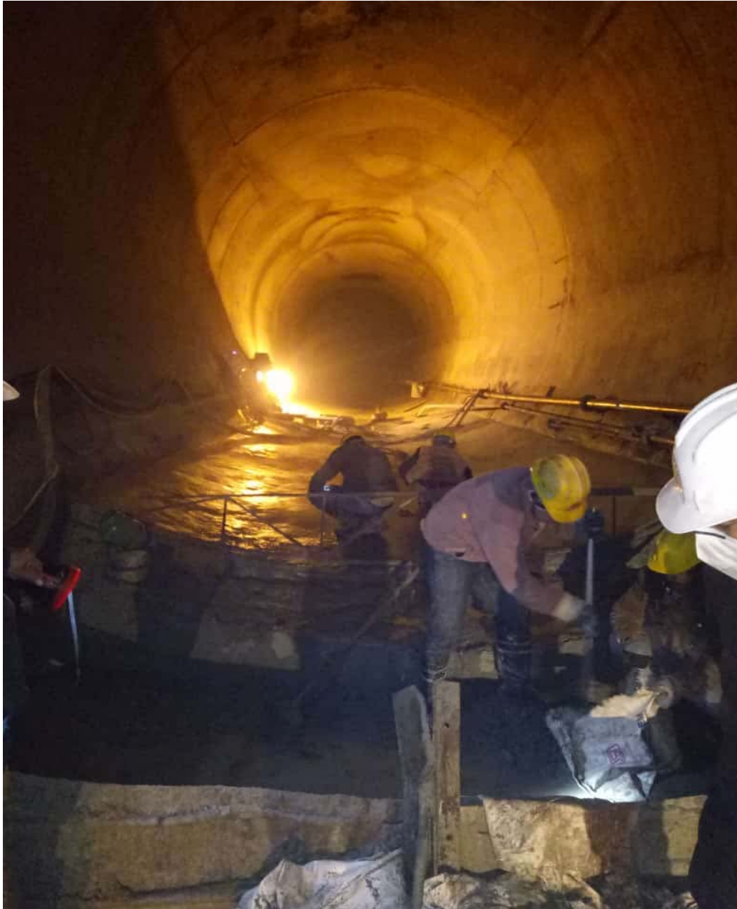
Figure 18: Manual Invert Concrete using template system
