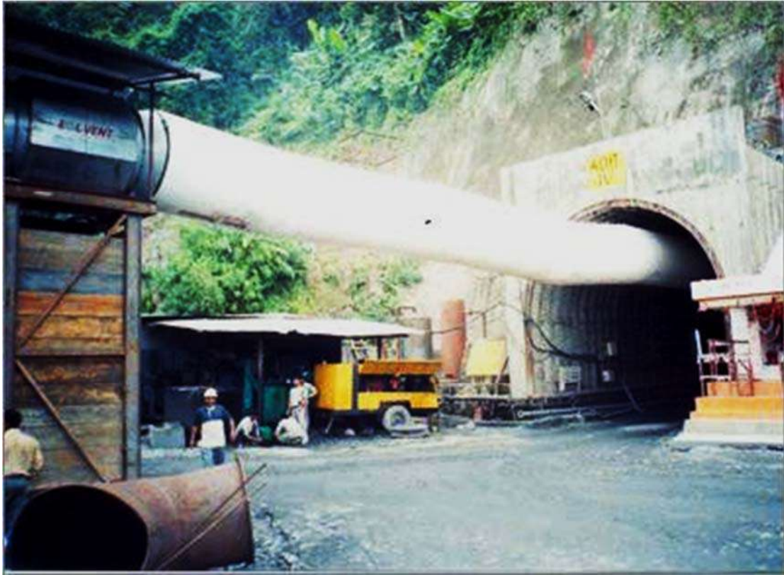
Figure 6: Defuming using Duct fans and connecting pipe
