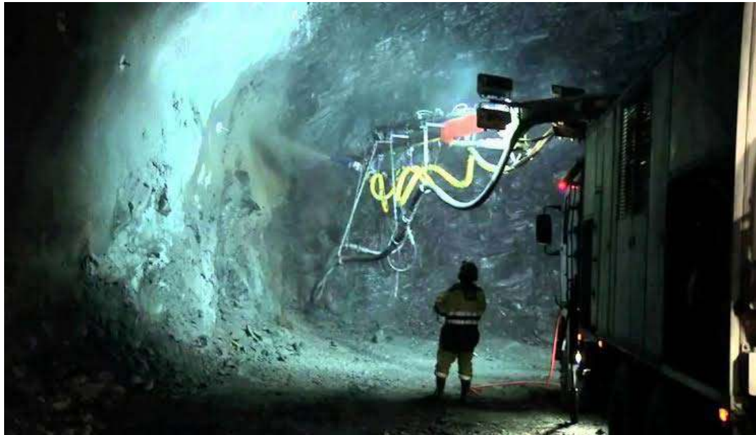
Figure 9: Shotcreting immediately after taking blast
