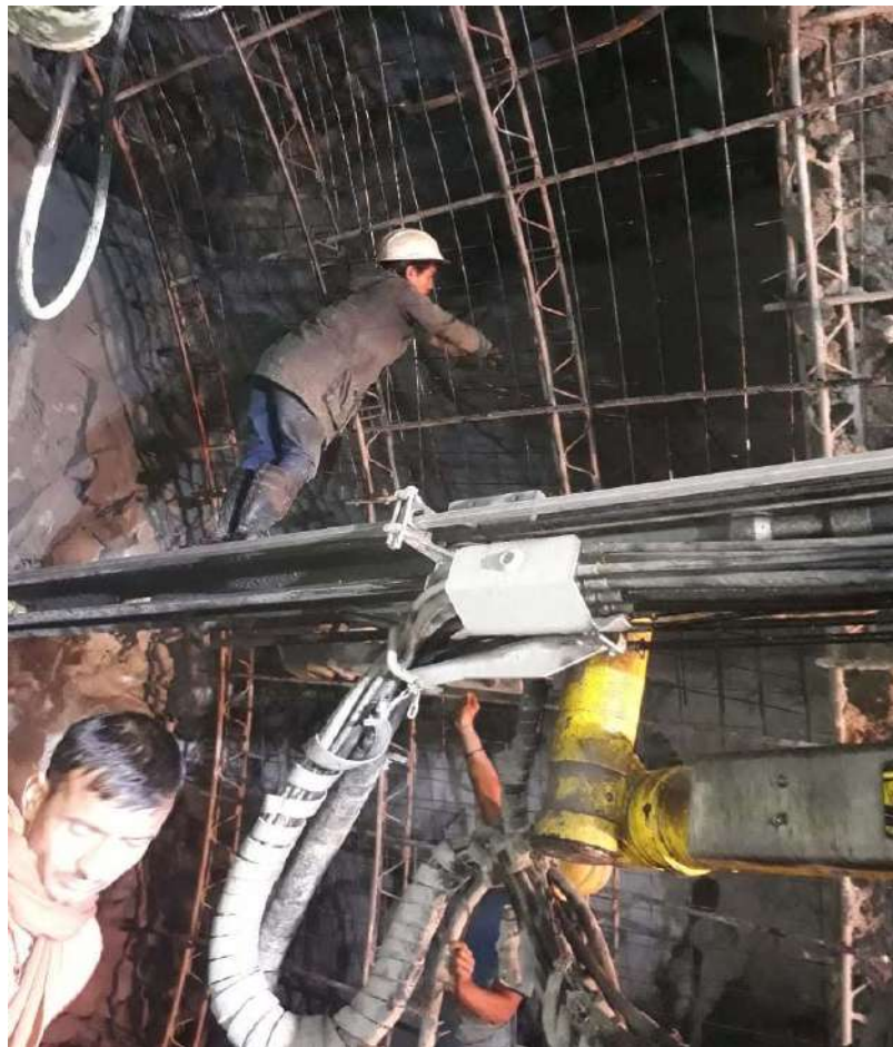
Figure 13: Installation of welded wire mesh
