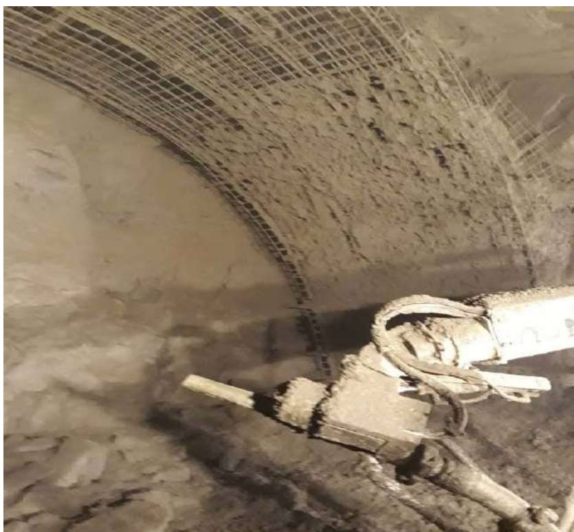
Figure 14: Final layer shotcrete
