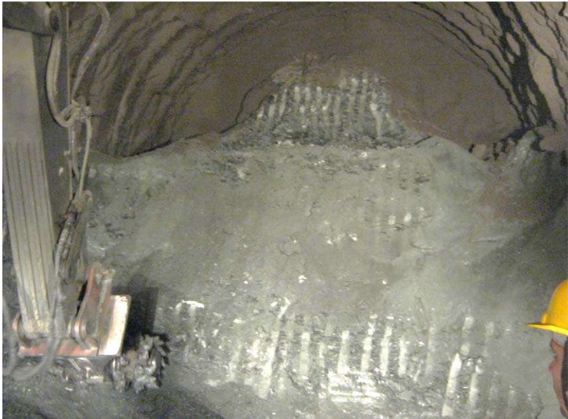
Figure 8: Excavation using Twin Cutter
