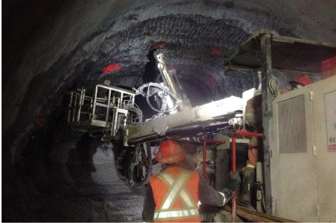
Figure 11: Rock bolts insertion using Boomer/Tamrock
