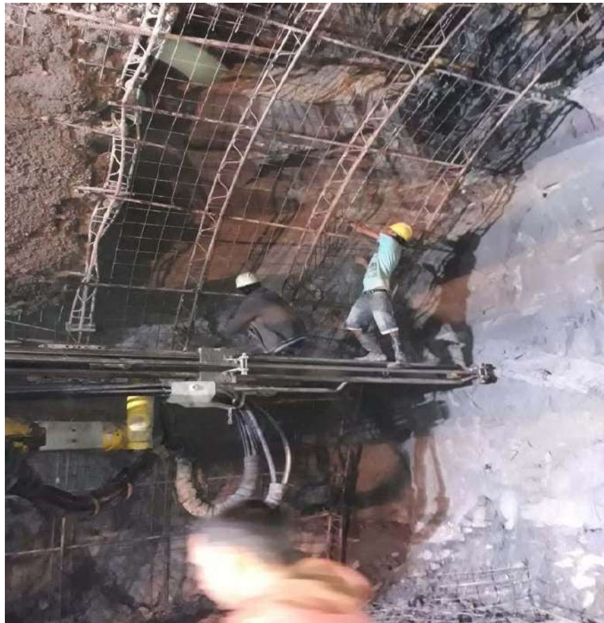
Figure 12: Lattice girder erection in Tunnel
