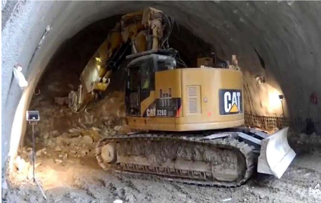
Figure 10: Mucking by Excavator
