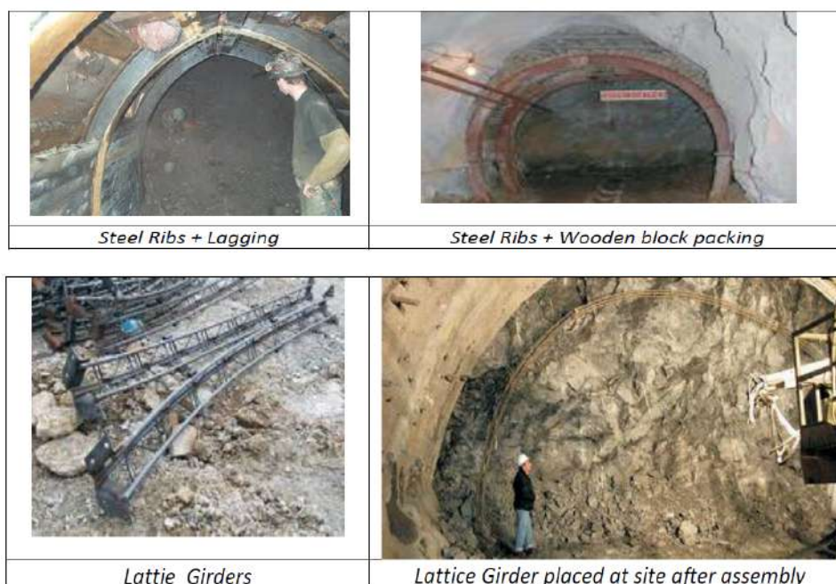
Figure 117 Shotcrete, steel ribs Lattice Girder
