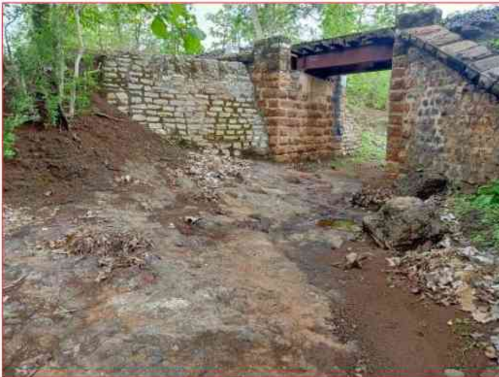
Figure 103 Rock exposure of Basalt is recorded at just below the culvert/minor bridge.
