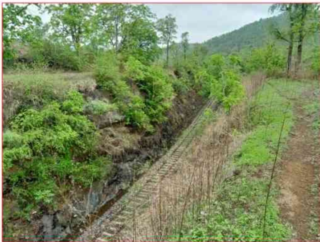
Figure 108 Exposure of compact, massive, fresh to slightly weathered Basalt rock exposed along railway cutting section.
