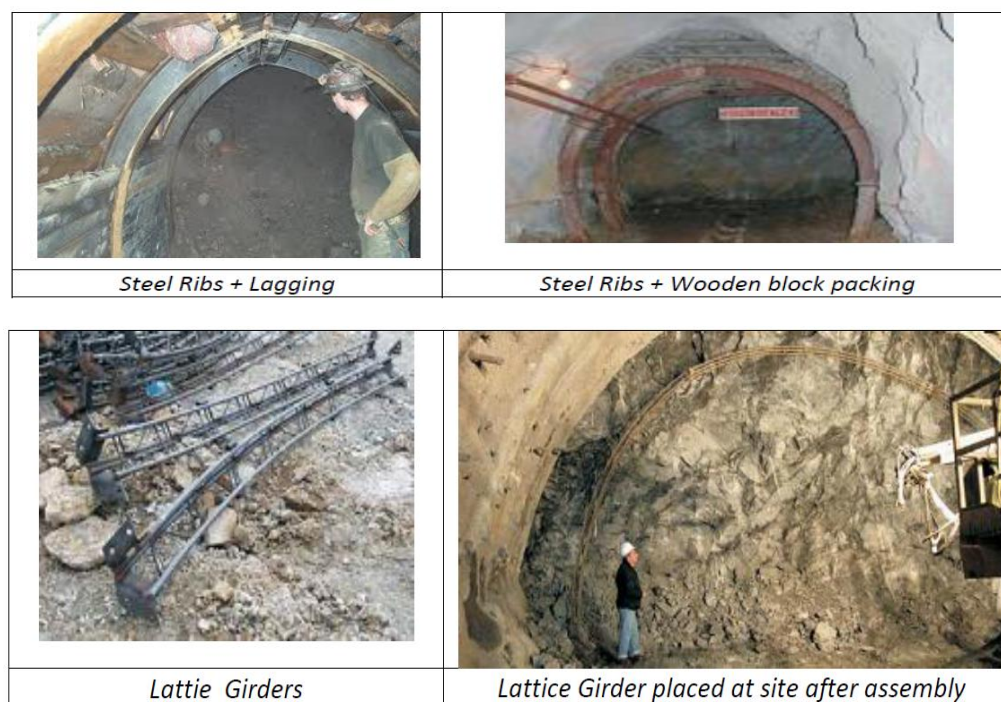
Figure 4 Shotcrete, steel ribs Lattice Girder
