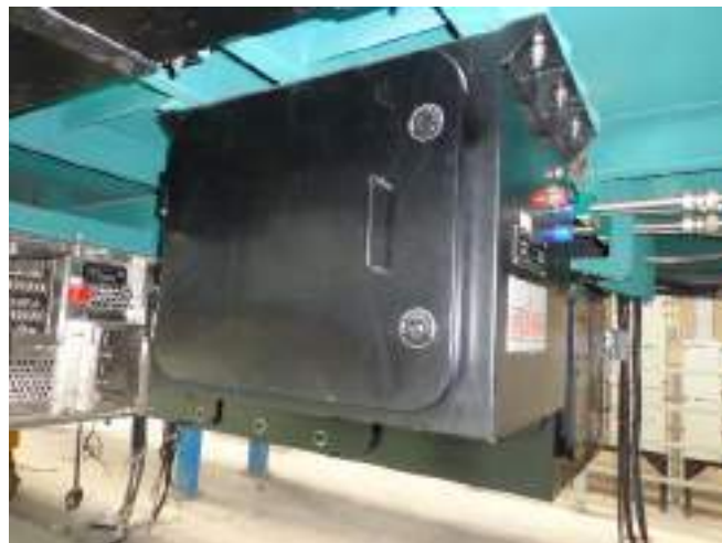
Figure 10: DC Link Earthing Switch
