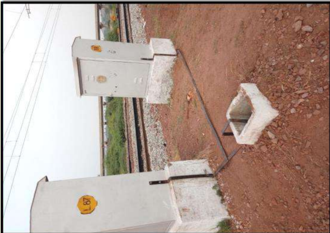
MS FLAT EARTHING AT LOCATION BOXES
